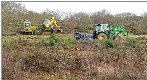
Diggers move in to prepare the scrape
